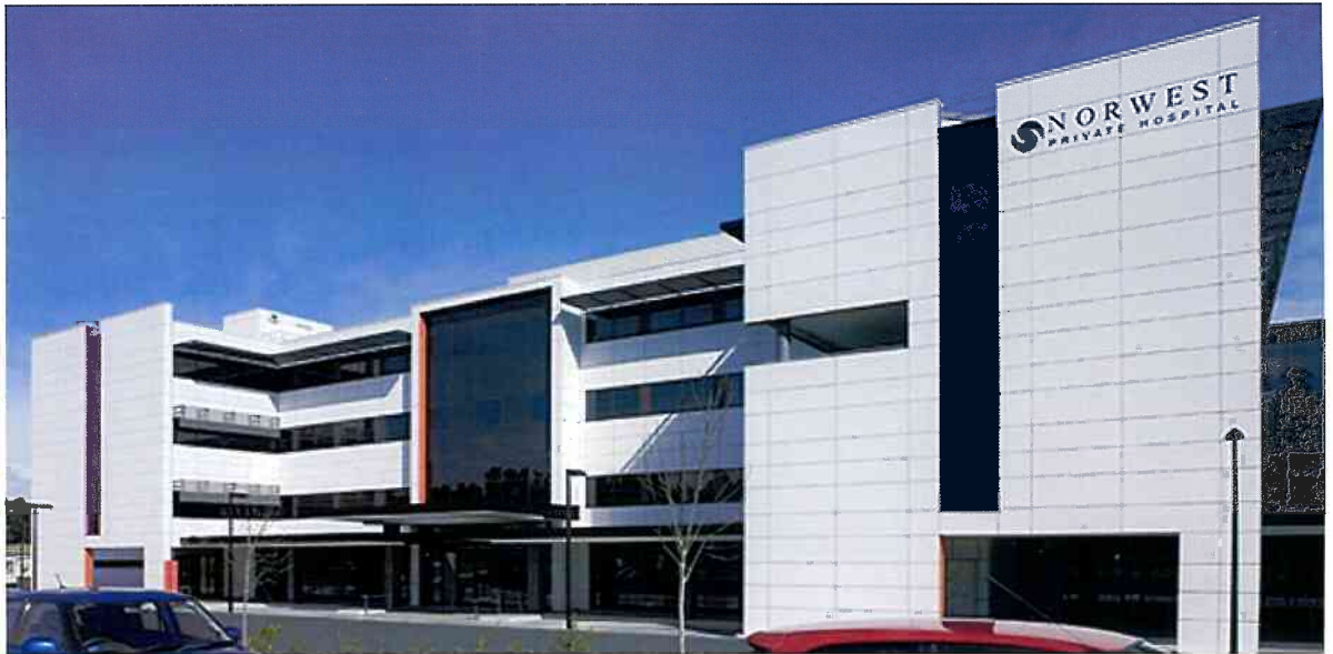
Norwest Private Hospital is located in Bella Vista and provides excellence in medical services and patient care to Western Sydney.
